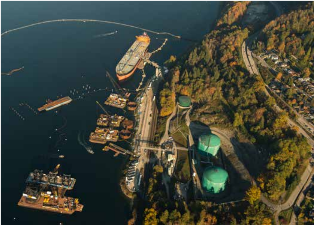
Kinder Morgan Westridge Marine Tanker Terminal at Burrard Inlet.
