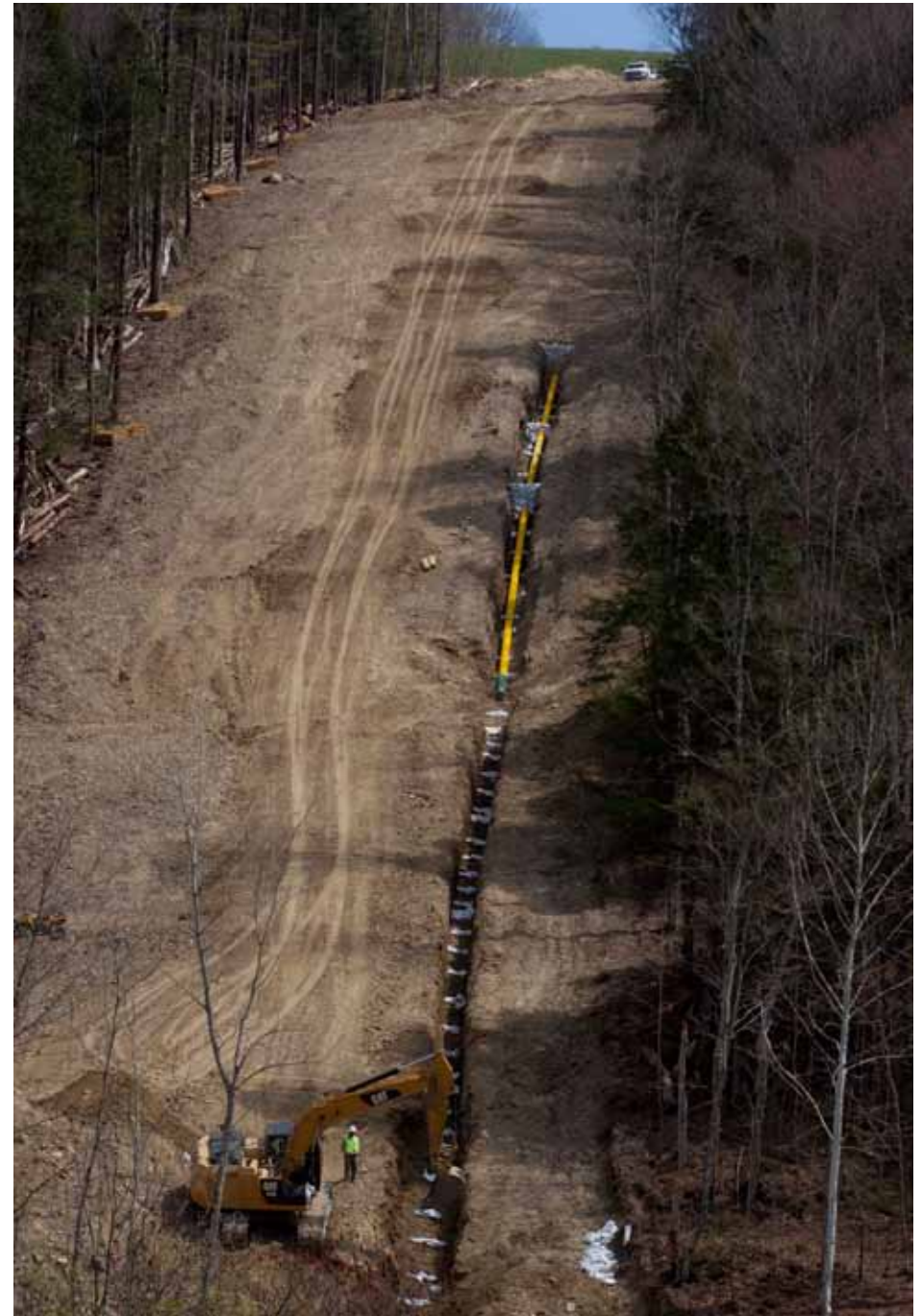
Pipelines being laid in Bradford County. Thousands of miles of pipeline are being laid around Pennsylvania to transport the gas.
